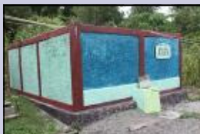
The Water Tank
